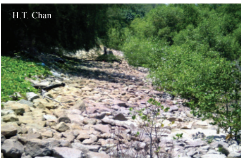
Fig. 13. Rock revetments constructed to safeguard against coastal erosion (L) Fig. 14. Sand-filled geotubes constructed to protect eroding shores (R)
